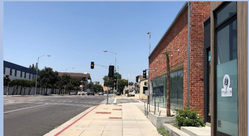
Sidewalk without landscaped buffer
